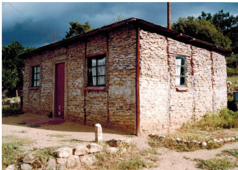
Fig. 4 Orthogonal building development – wattle lath and packed stone (Photo: Author 2002)
